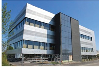
mRNA Manufacturing (mMC) facility
