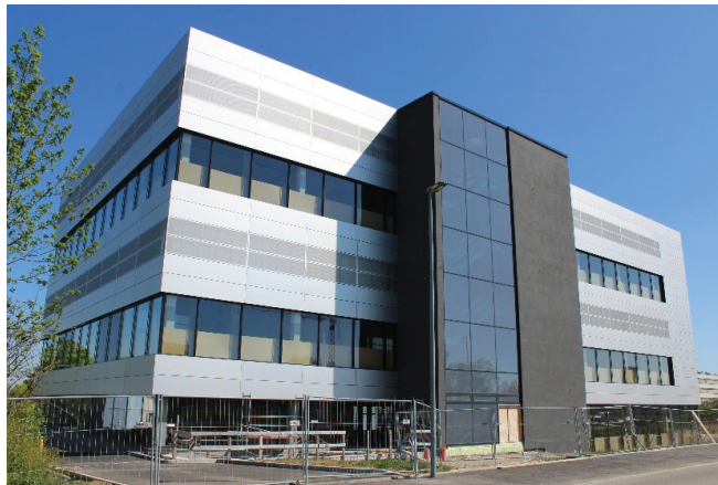
GMP IV facility
